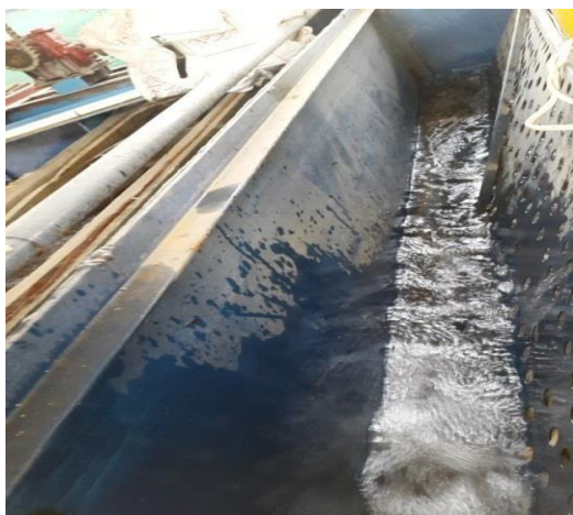
Figure :3.5 (e) Stilling Chamber
